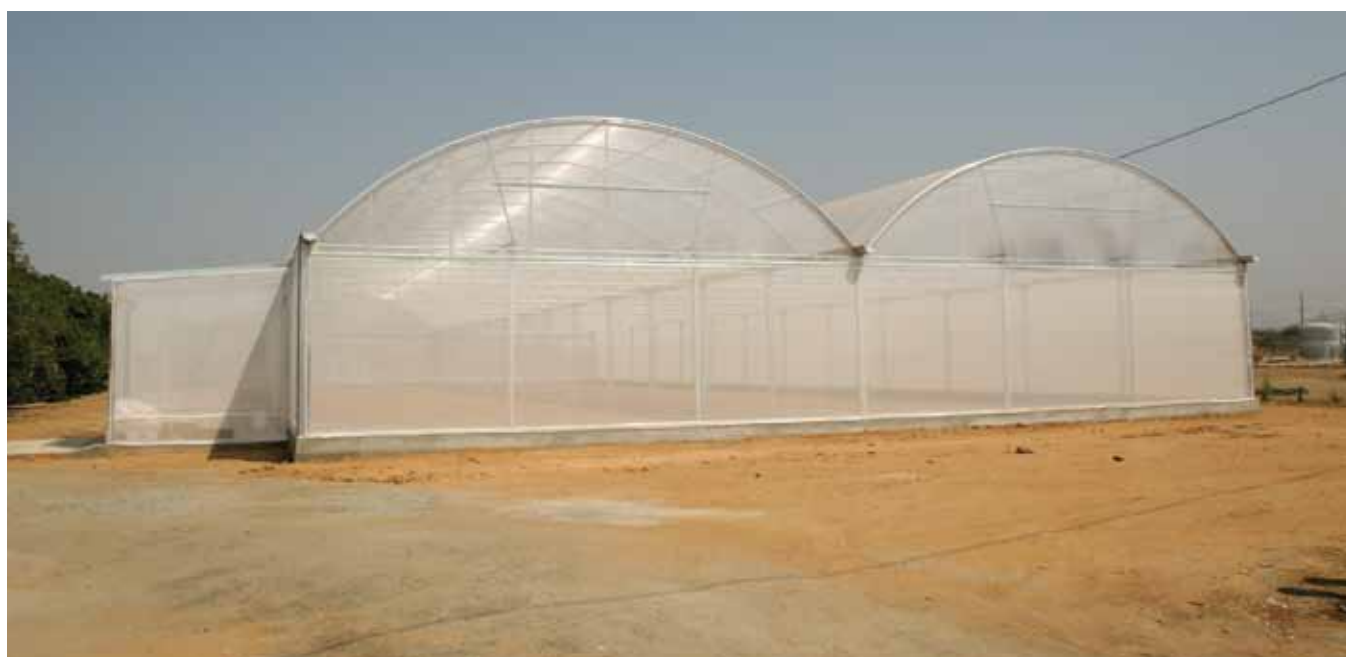
Screenhouse for registered (mother) trees. All registered budwood source trees in California were required to be grown in approved protected structures starting Jan. 1, 2012.
